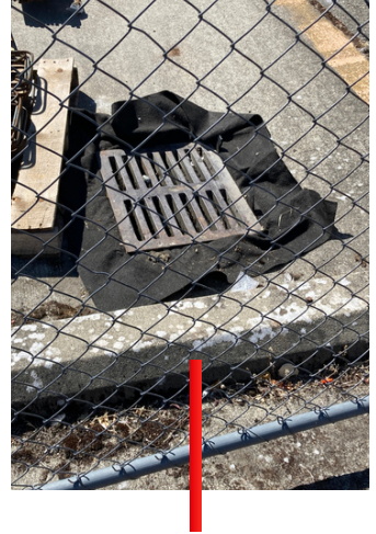
Sufficient sediment control
