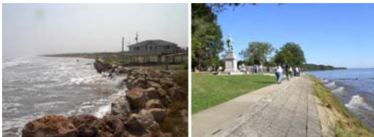
Figure 4-3 Two types of stone revetments (a) near Surfside, Texas and (b) at Jamestown, Virginia. Copyright Risingsea.net (2009). Used by permission.
