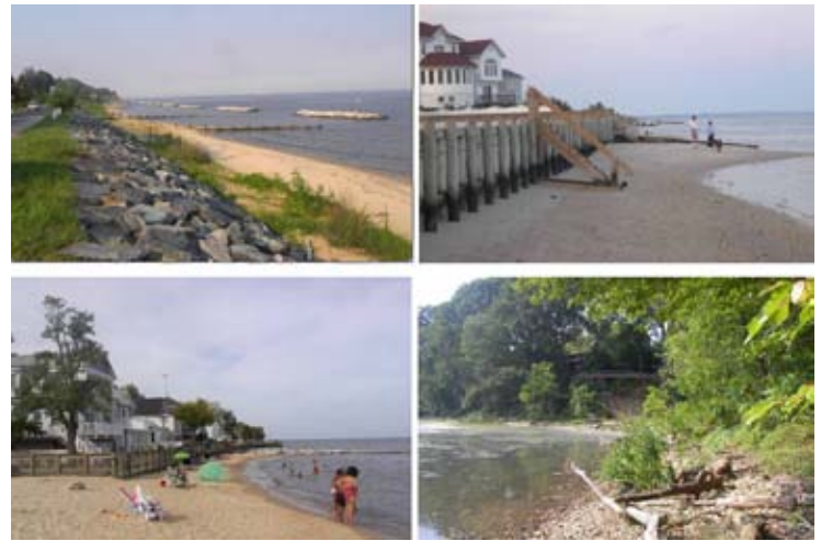
Figure 4-6 Hybrid approaches to shore protection. (a) Breakwaters and groins along Chesapeake Bay in Bay Ridge (near Annapolis) Maryland [July 2008]. The rock structures parallel to the shore in the bay are breakwaters; the structures perpendicular to the shore are groins; (b) wooden groins and bulkhead along the Peconic Estuary on Long Island, New York [September 2006]. The beach is wider near the groin and narrower between groins; (c) a nourished beach with a terminal groin at North Beach, Maryland [September 2008] (d) a dynamic revetment placed over the mud shore across Swan Creek from the Fort Washington (Maryland) unit of National Capital Parks East. Logs have washed onto the shore since the project was completed [July 2008]. Copyright Risingsea.net (2009). Used by permission.
