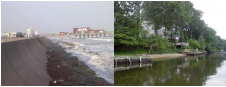
Figure 4-2 Seawalls and Bulkheads (a) Galveston Seawall in Texas [May 2003] and (b) Bulkheads with intervening beach along Magothy River in Anne Arundel County, Maryland [August 2005]. Copyright Risingsea.net (2009). Used by permission.
