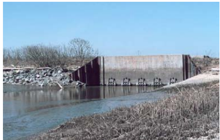
Figure 4-5 The tide gate at the mouth of Army Creek on the Delaware side of the Delaware River. The tide gate drains flood and rainwater out of the creek to prevent flooding. The five circular mechanisms on the gate open and close to control water flow (Source: NOAA Photo Library).
