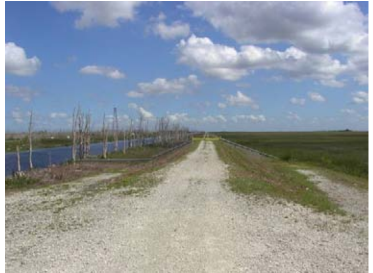
Figure 4-4 A dike in Miami-Dade County, Florida. Copyright Risingsea.net (2009). Used by permission.
