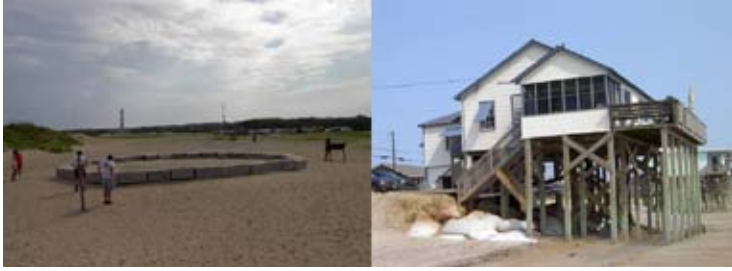
Figure 4-7 Relocating Structures Along the Outer Banks (a) Cape Hatteras Lighthouse after relocation at the Cape Hatteras National Seashore, Buxton, North Carolina [June 2002]. The original lighthouse location is outlined in the foreground, and; (b) A home threatened by shore erosion in Kitty Hawk, North Carolina [June 2002]. The geotextile sand bags are used to protect the septic system. Copyright Risingsea.net (2009). Used by permission.
